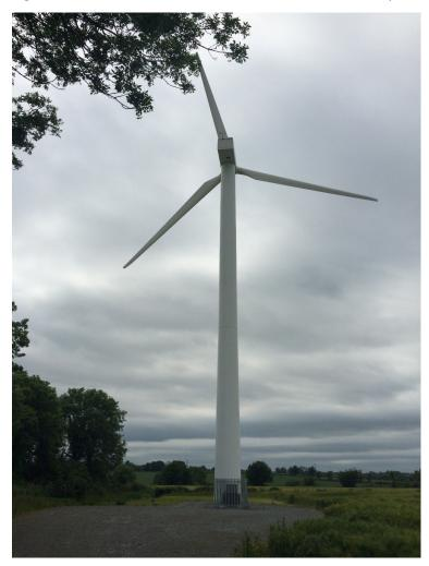
Figure 21: Vestas V44 wind turbine 600 kW at Balrath, County Meath
